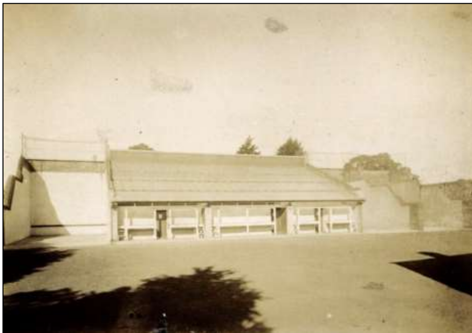
Three of the courts roofed and enclosed in 1906
